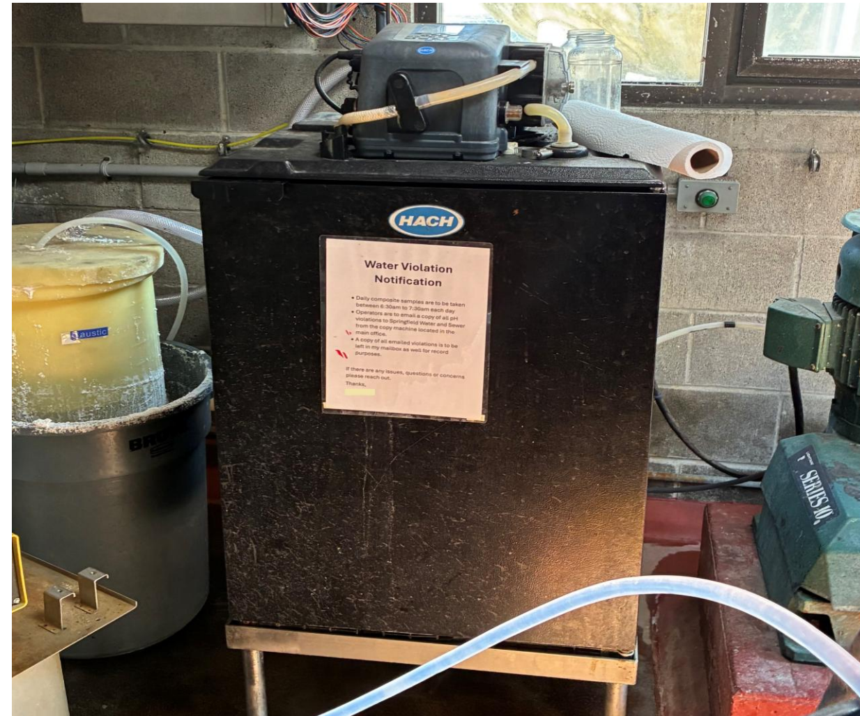
Facility's auto sampler
